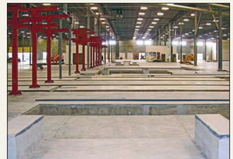
PRATT INDUSTRIES (U.S.A.) INC. – FORT WORTH, TX
