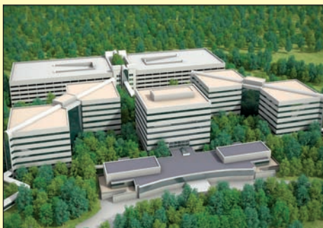
Following Cadence McShane's renovation of the former five-building, 1.2 million square foot HP office campus for Lone Star College (LSC), the firm was retained to complete 66,500 square feet of additional classroom construction at the LSC – University Center at University Park campus.
