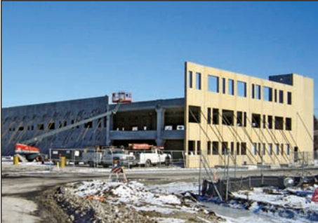
RANDHURST VILLAGE PARKING GARAGE – MT. PROSPECT, IL
