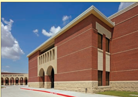
Plano ISD recently opened the new $35.3 million, 282,000 square foot McMillen High School in Murphy, Texas, welcoming 1,100 students to its 2011-12 inaugural school year following Cadence McShane's on-time completion of this sizable, two-story educational campus.
