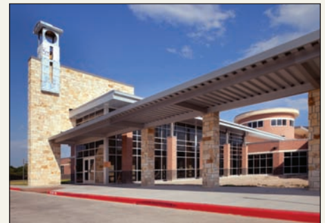
EDGEWOOD ELEMENTARY SCHOOL – HOUSTON, TX
