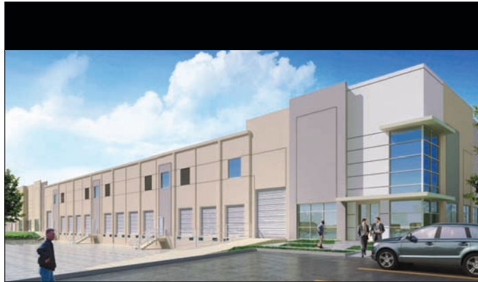
Cadence McShane has been selected by developer, The Carson Companies, to construct the Sens Road Distribution Center, a new 267,280 square foot multi-tenant industrial facility in La Porte, Texas, offering direct access to both Barbour's Cut and the new Bayport Container and Cruise Terminal.
