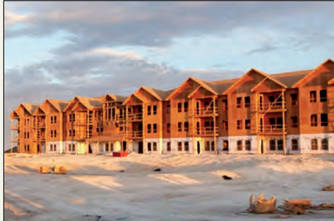
LAS BRISAS MANOR SENIOR APARTMENTS – DEL RIO, TX
