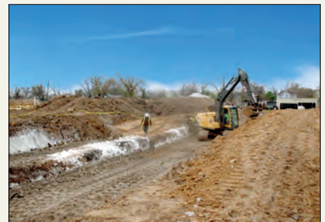
ATHERTON ELEMENTARY SCHOOL – HOUSTON, TX
