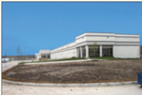
CLAYPOINT DISTRIBUTION PARK – HOUSTON, TX
